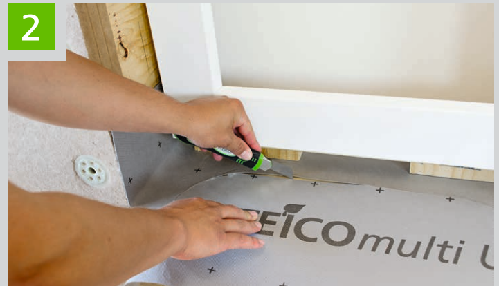
The windows are installed on the underlay. Before installing insert space between STEICOfix and cut the underlay back trapezoidally (see picture 5)
