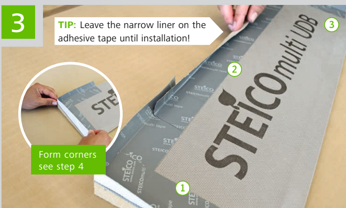
Then apply the STEICOmulti tape F 20/40 mm adhesive strips to the insulating wedge in such a way that a three-sided "trough" is formed
